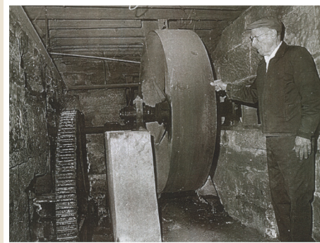
Water power turned simple wheels and gears, like these shown with Mack Elson, operating a complex system of milling equipment.
